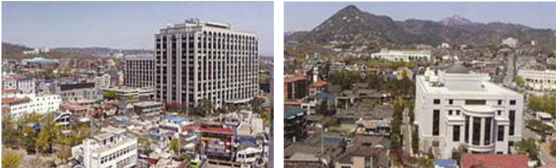
Figure 4.7 The Traditional and modern environment of Bukchon District
