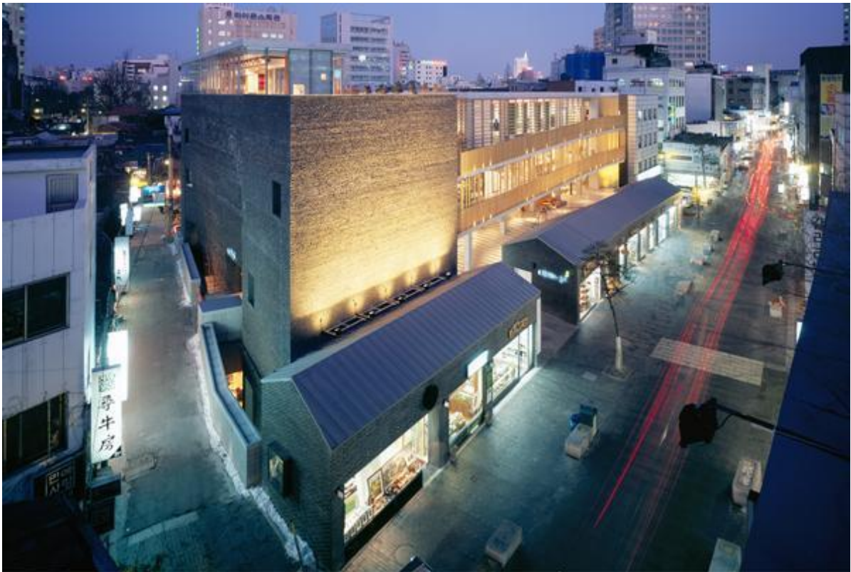
Figure 5.7 The outside of new craft building built on the site of the twelve small shops
