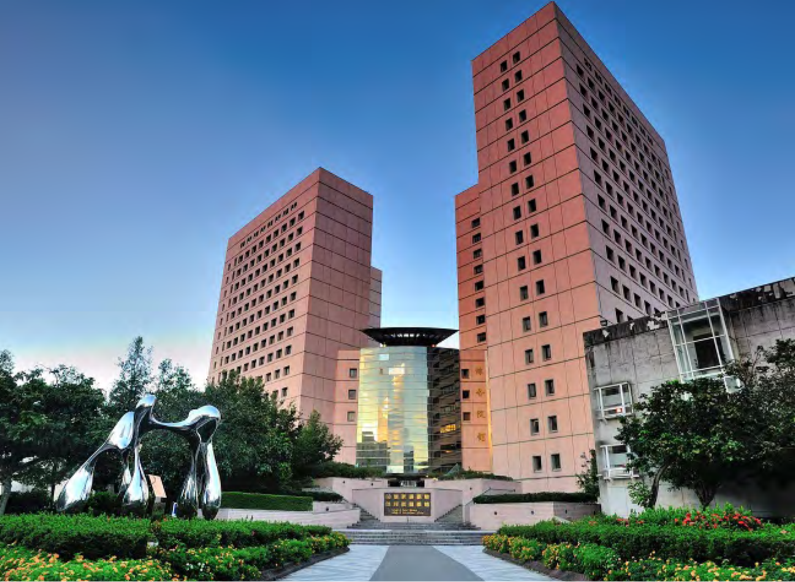
▲ General building of colleges
